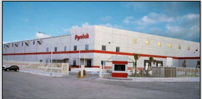
Pyrotek's new production and warehouse facility in Apodaca, Mexico
